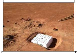
When installing WHITE base plate, the four rectangular areas in base anchor must be clear of dirt, allowing for insertion of base plate.
